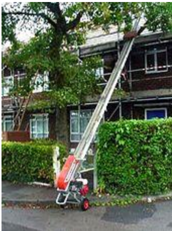
Builder's hoist, with small gasoline engine
